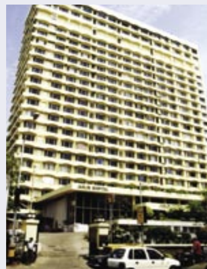
Jaslok Hospital, Mumbai.
